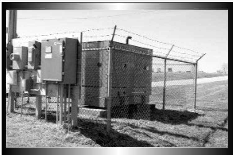
Generator & Control Panel.
