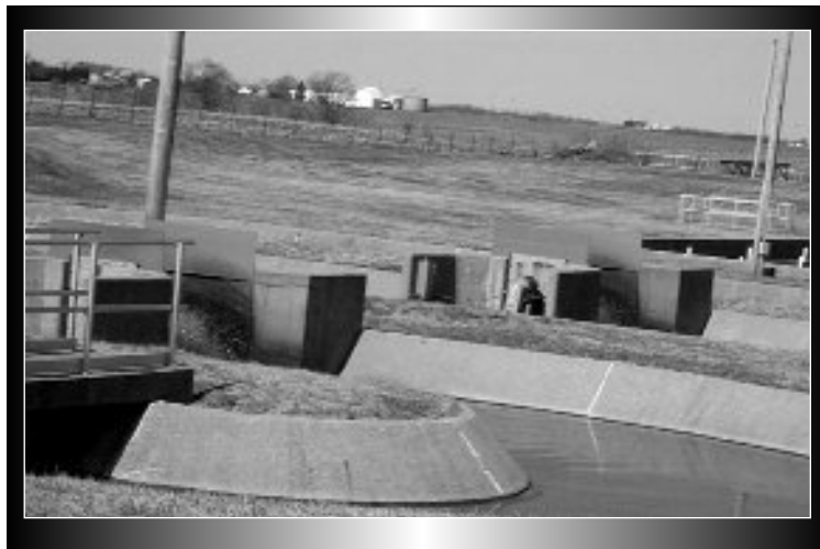
Twin oxidation ditches
