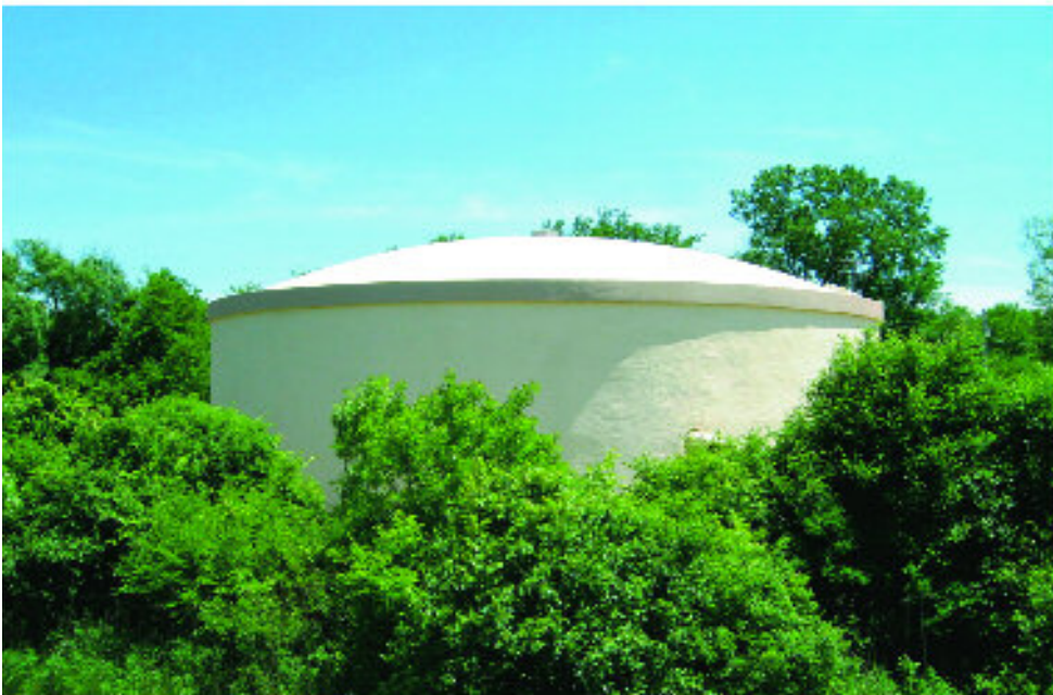
1.0 MG Natgun water tank for the Village of Roson, IL. Engineering by Robinson Engineering, Ltd., South Holland, IL.
