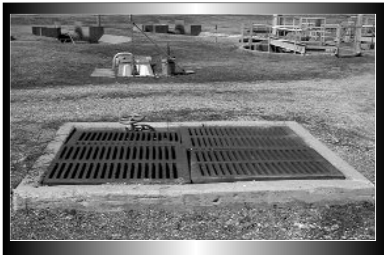
Diversion chamber at WWTP
